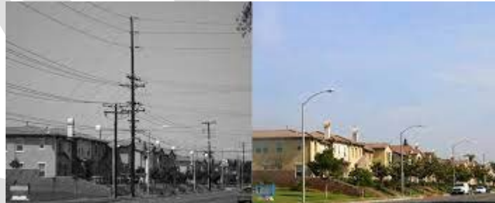
Example of Relocated Powerlines
