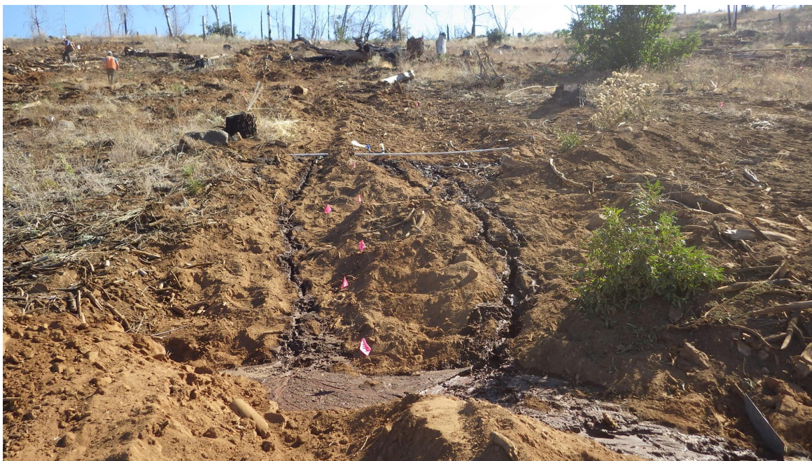
Water bar spacing set to 1/2 the prescribed distance (15 m), or double the frequency: " Double-drainage "
