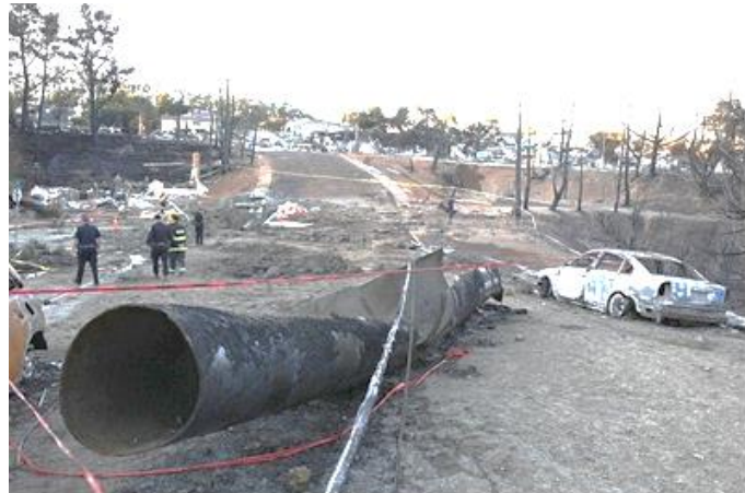
Figure 67: San Bruno Pipeline Explosion
