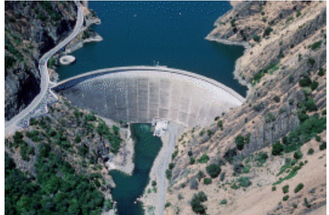
Monticello Dam – Napa County, CA
