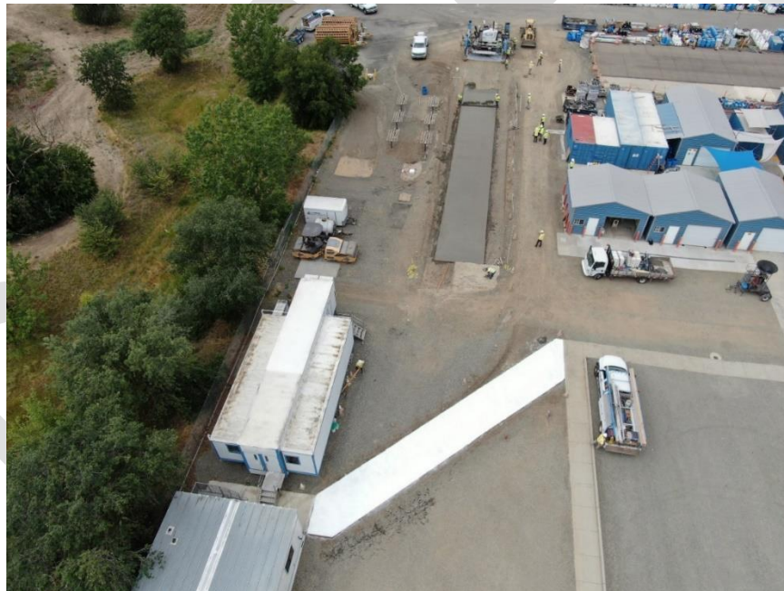
944 Figure 21. Location of test sections (white path at the bottom of the picture; picture taken after 945 the application of the curing compound on the lean concrete base).
