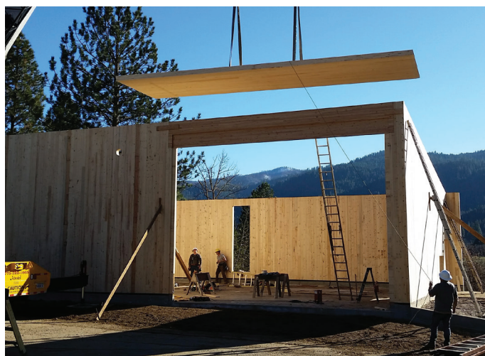
CLT building in construction in Quincy
