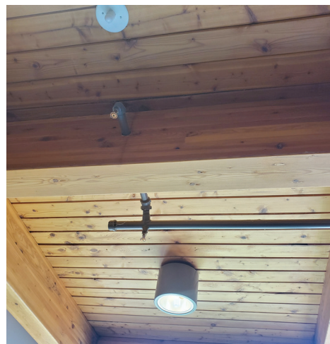
Mass timber buildings outfitted with sprinklers for fire events makes the material appropriate for use in dense urban areas
