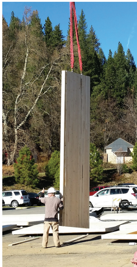
A CLT panel gets lifted into place at the construction site
