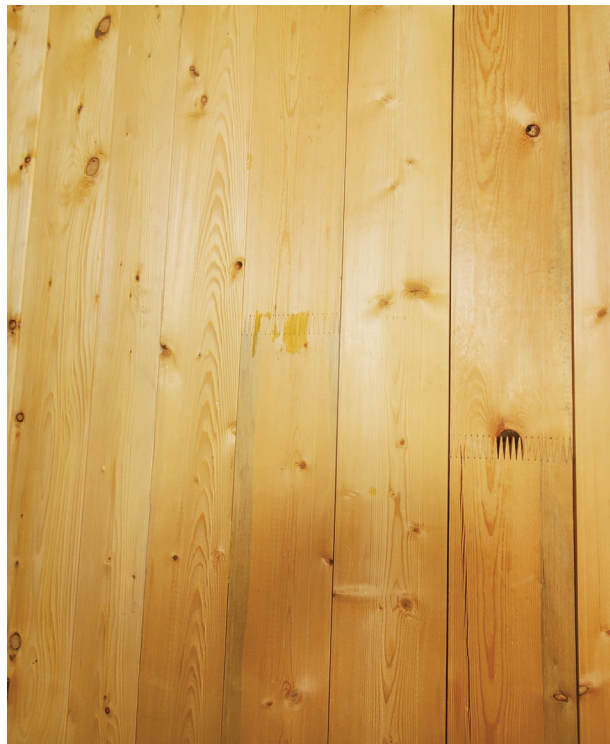
A CLT wall with finger joints
