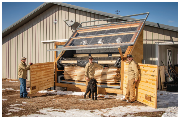
A solar kiln to dry lumber to desired moisture content for CLT fabrication (photo courtesy of TimberAge Systems)
