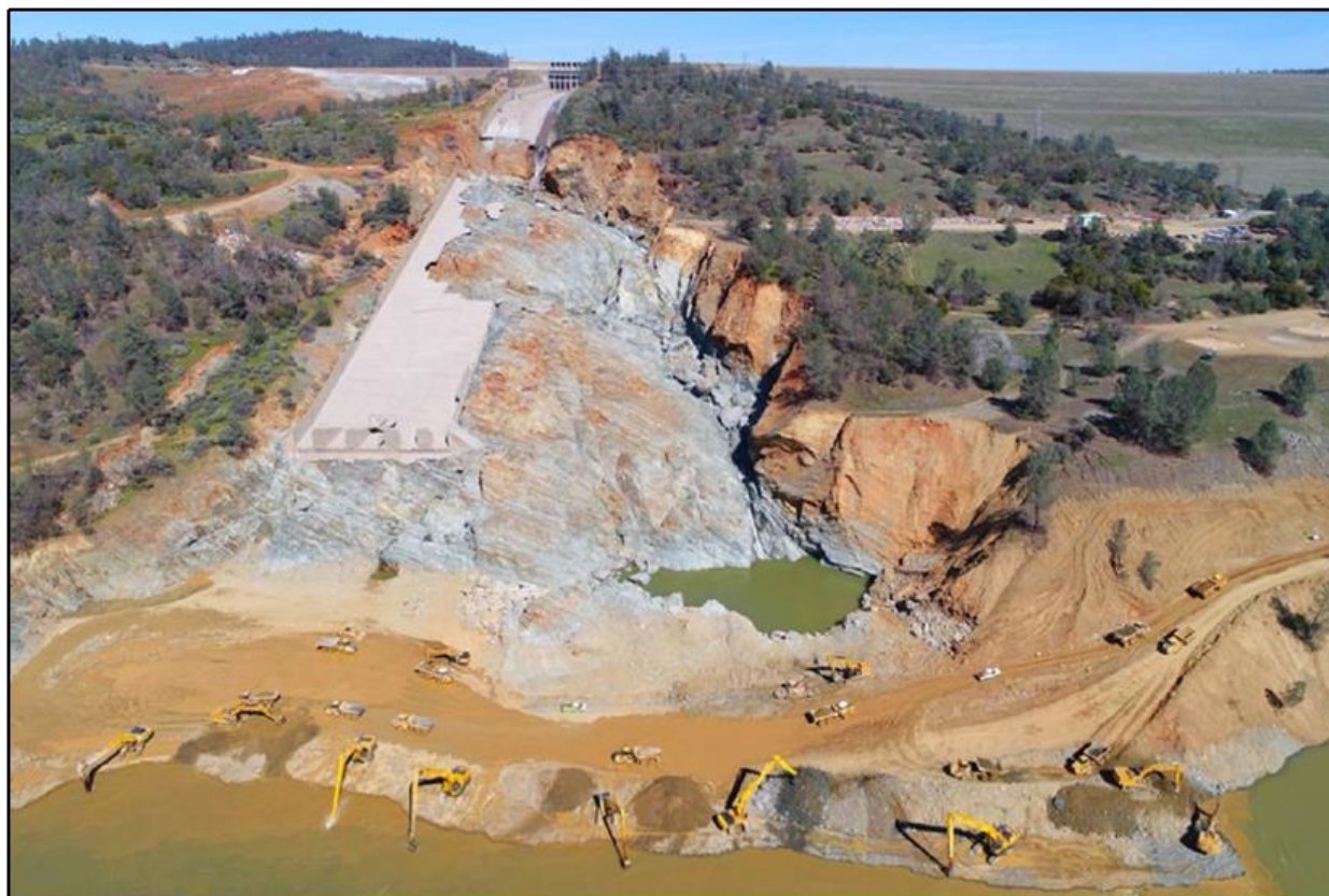
Figure 4-28 Ultimate Damage at Oroville Dam Spillway
