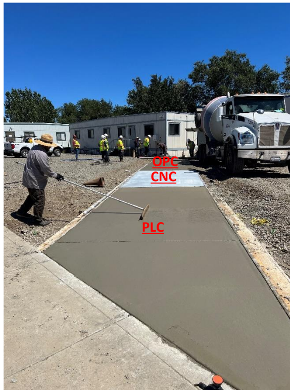
1069 Figure 29. Trowel finishing of PLC section (bottom of photograph); CNC section already 1070 sprayed with curing compound (middle of photograph; note that white covering is from the 1071 curing compound and not the CNC effect); rolling screed consolidation of OPC concrete 1072 (middle-top of photograph).
