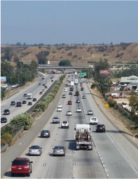
Interstate 10 is the primary source of noise and vibration in southwest Yucaipa.
