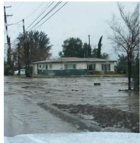
The 2010 flash floods damaged roadways and homes in Yucaipa.
