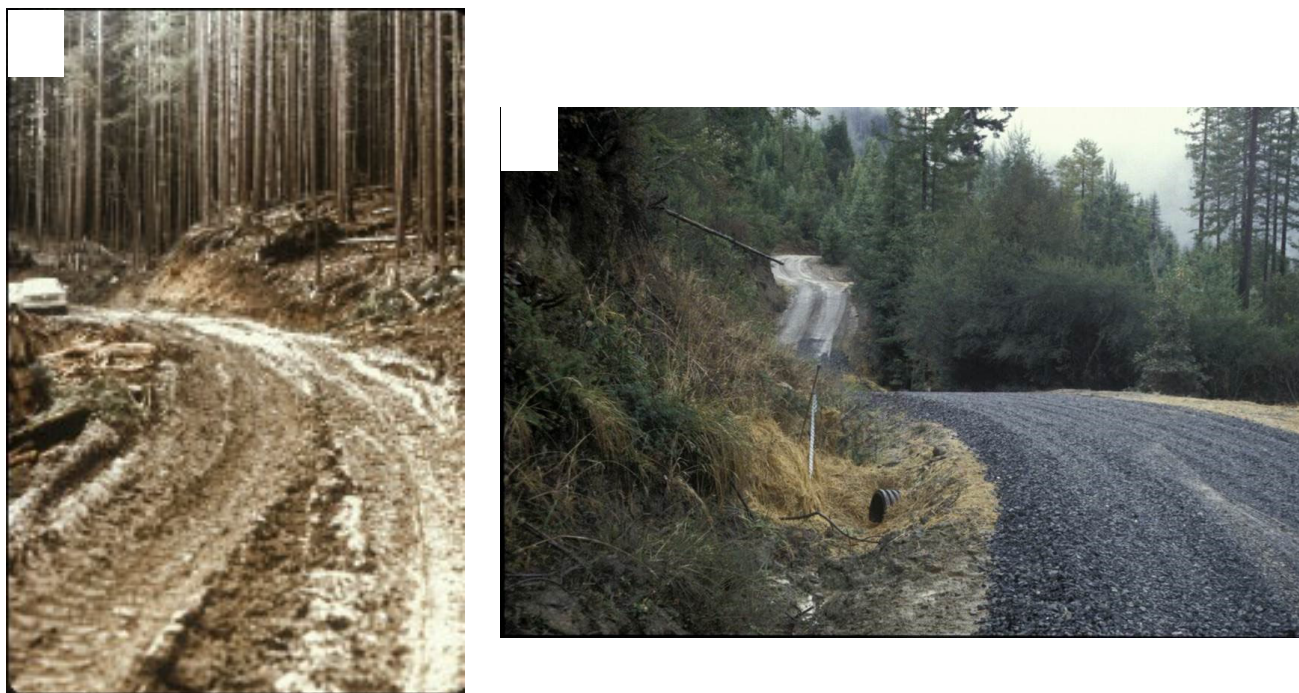
Figure 6. a) Photo of a primary road used for timber hauling in about 1990, and b) the same road in 2001 after upgrading by rocking and improved drainage.
