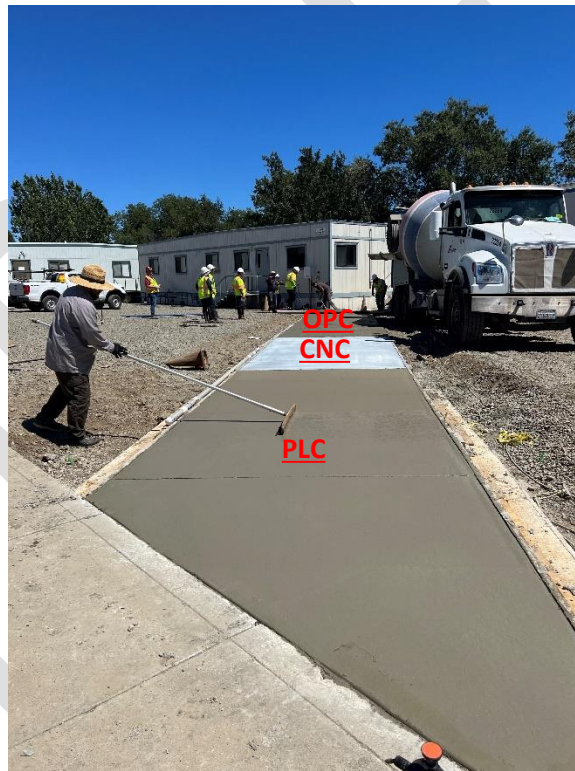
1067 Figure 29. Trowel finishing of PLC section (bottom of photograph); CNC section already 1068 sprayed with curing compound (middle of photograph; note that white covering is from the 1069 curing compound and not the CNC effect); rolling screed consolidation of OPC concrete 1070 (middle-top of photograph).
