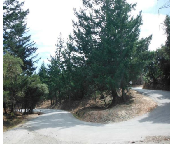
Figure 4. San Mateo County – Mechanized – After
