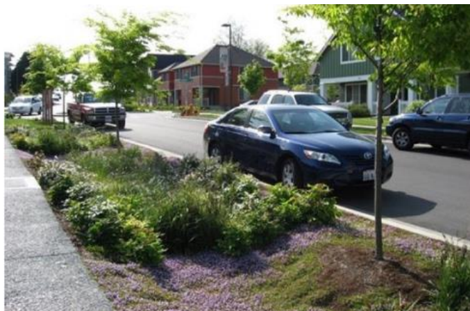
Green Infrastructure: Bioswale
