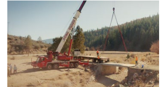
Figure 1. Bridge constructed using CNCs from woody biomass, Yreka, CA.
