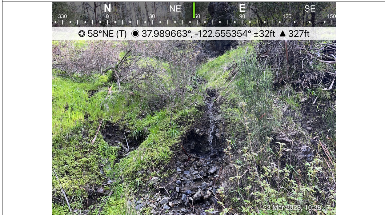
Photo 6. Aquatic drainage feature observed flowing through project area. (Reconnaissance Survey, 3/23/2023)
