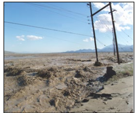
Flooding along Indian Canyon Drive, January 11, 2005.
