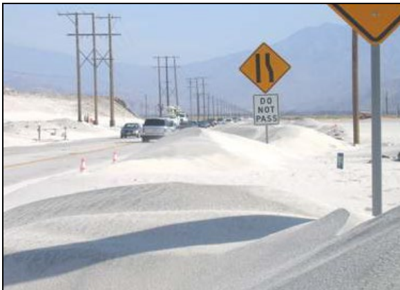
Windblown sand hazard along Indian Canyon Drive.
