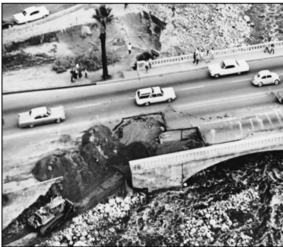
Flood damage to Highway 111 from 1965 storms.
