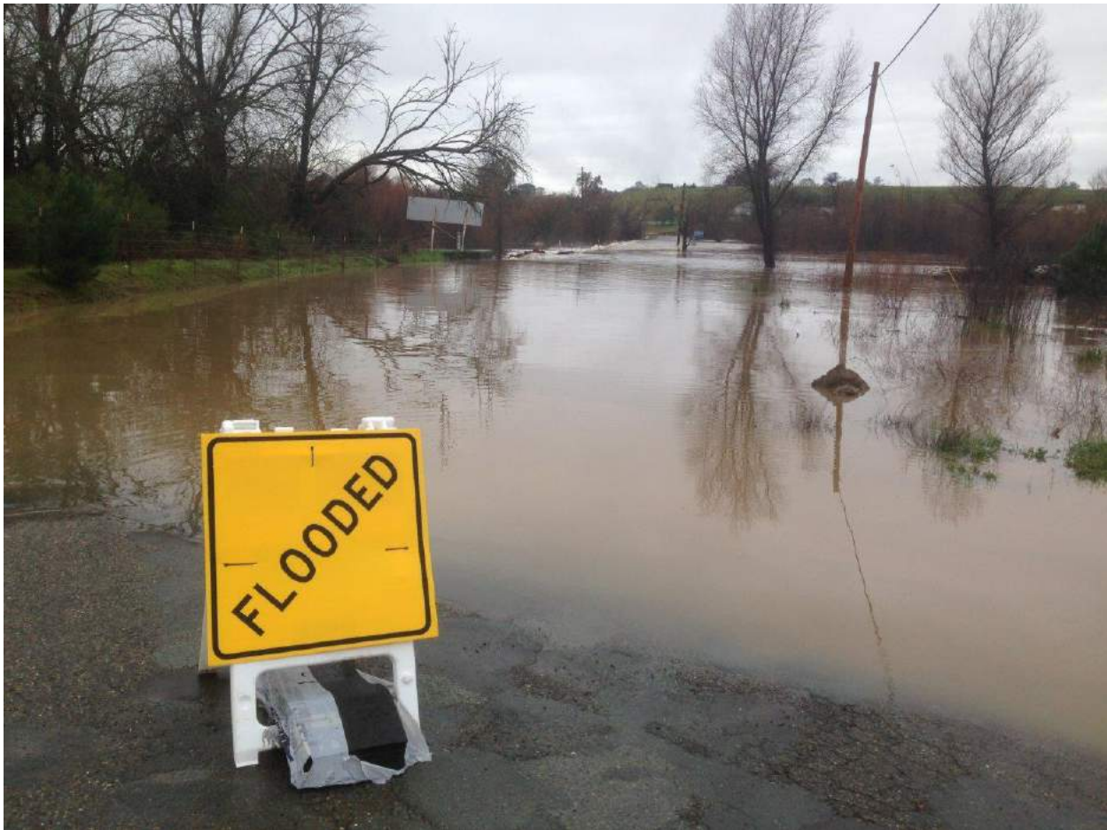
Figure 4-53 Amador County 2017 Flooding
