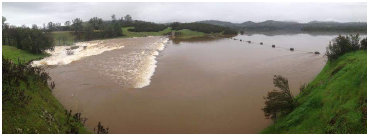
Figure I-6 Spillway Overtopping in 2017
