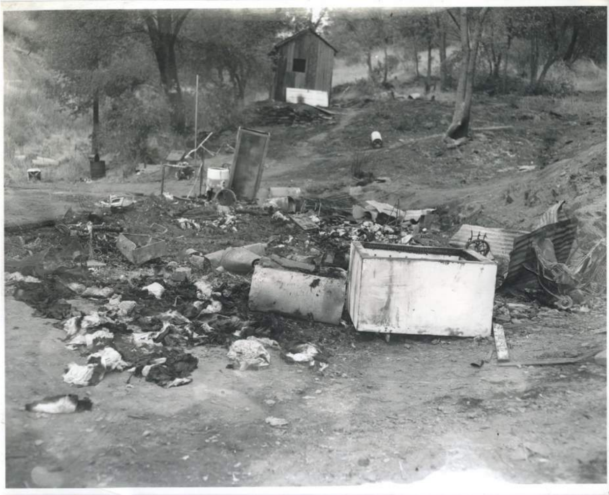
Figure 4-76 Rancheria Creek Fire Damages
