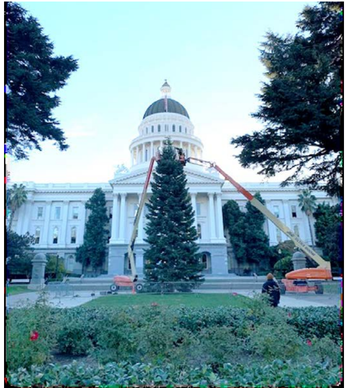
Figure 1. The Capital Christmas Tree being installed on November 4.
