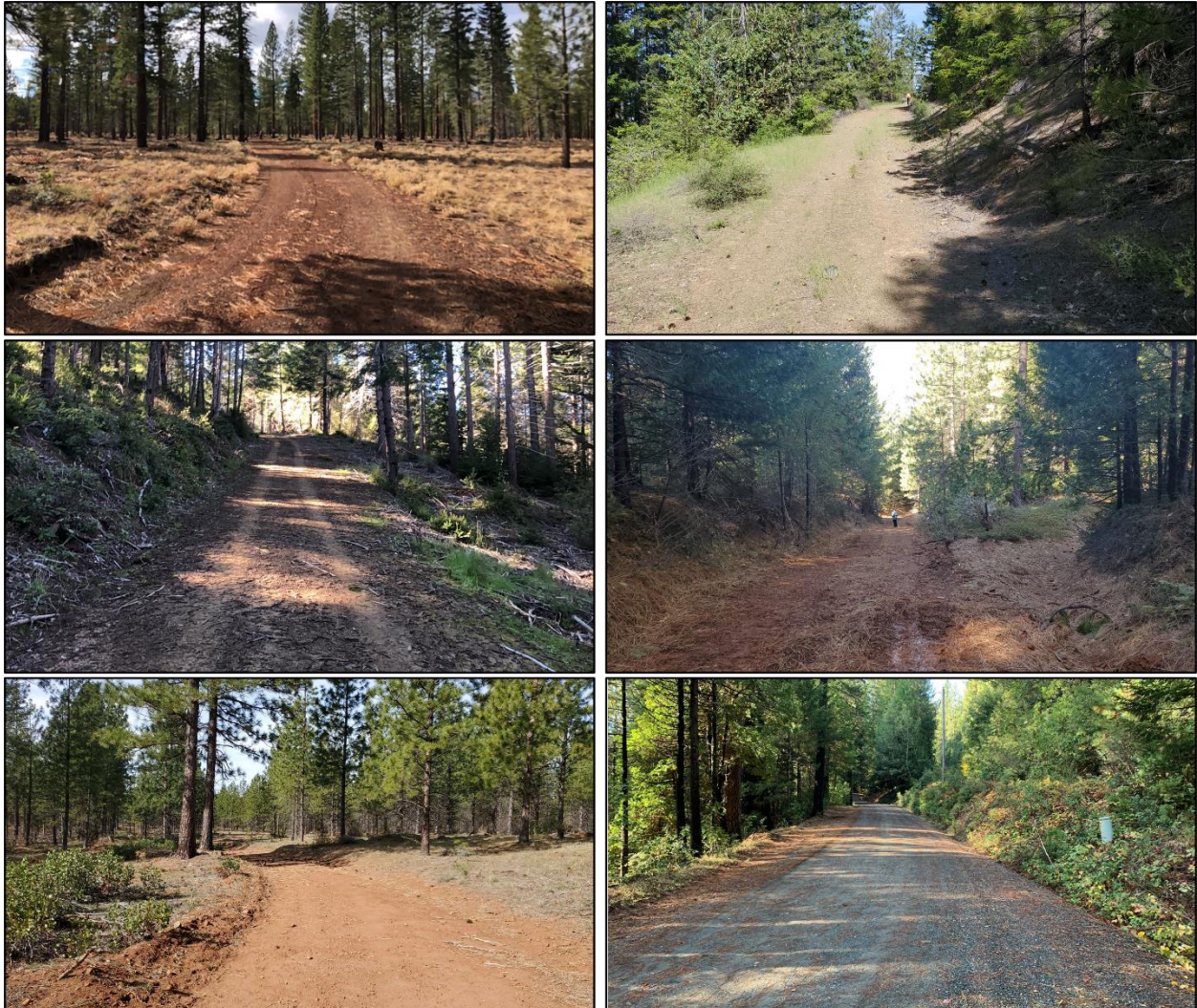
Figure 16: Examples of sampled roads on Industrial timberland FFP Notices. All roads shown are native surface seasonal roads, with the exception of the bottom right photo which is a rocked permanent road.
