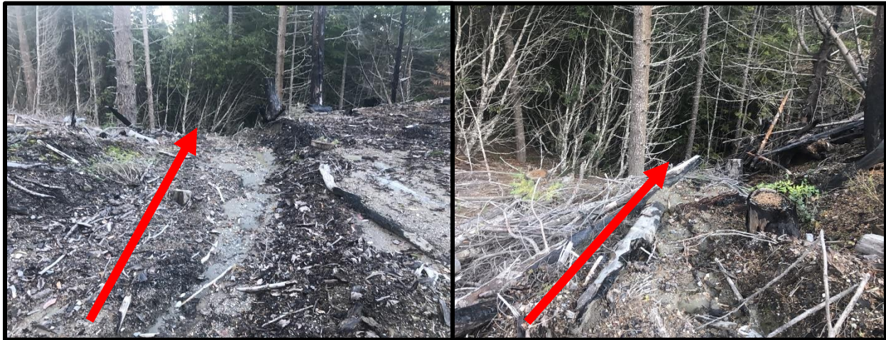
Figure 22: A dry ford Class III crossing that resulted in a sediment discharge in excess of one yard 3 , in the Coast FPA. Red arrows indicate direction of runoff and sediment delivery.
