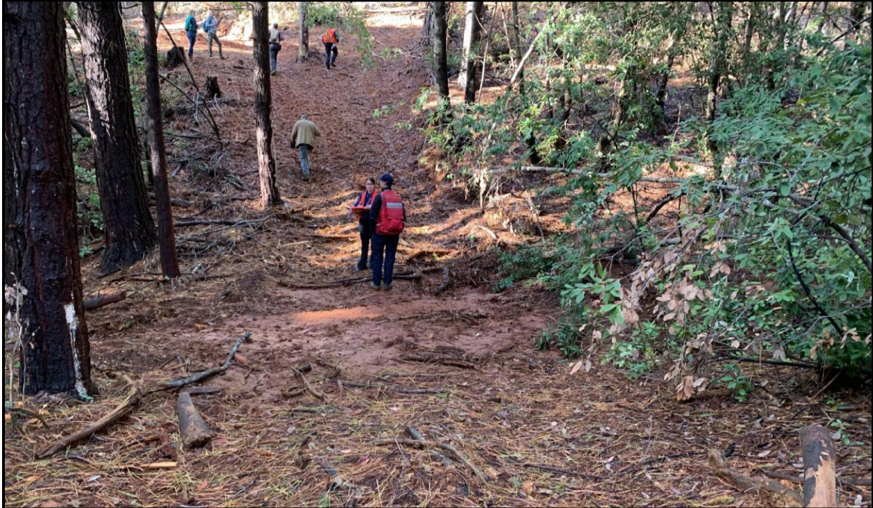
Figure 26: A Class III tractor crossing that was unmapped on a mapped Class III watercourse, with extended approach lengths a sediment discharge over one yard 3 .
