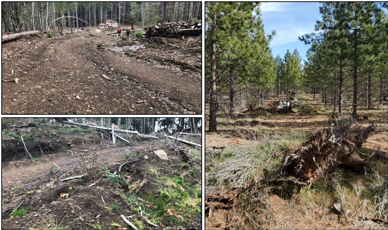
Figure 19: Open and actively used (not abandoned) temporary roads in the Coast FPA (top and bottom left) with visible road surface and drainage rills present, and a temporary road that was abandoned in the Cascade FPA (right).
