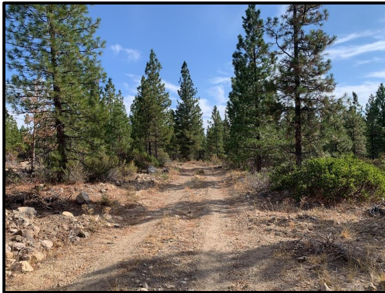
Figure 14: A native surface road within an FFP Notice on Industrial timberland that was less than 5% in slope and on generally flat hillslopes.
