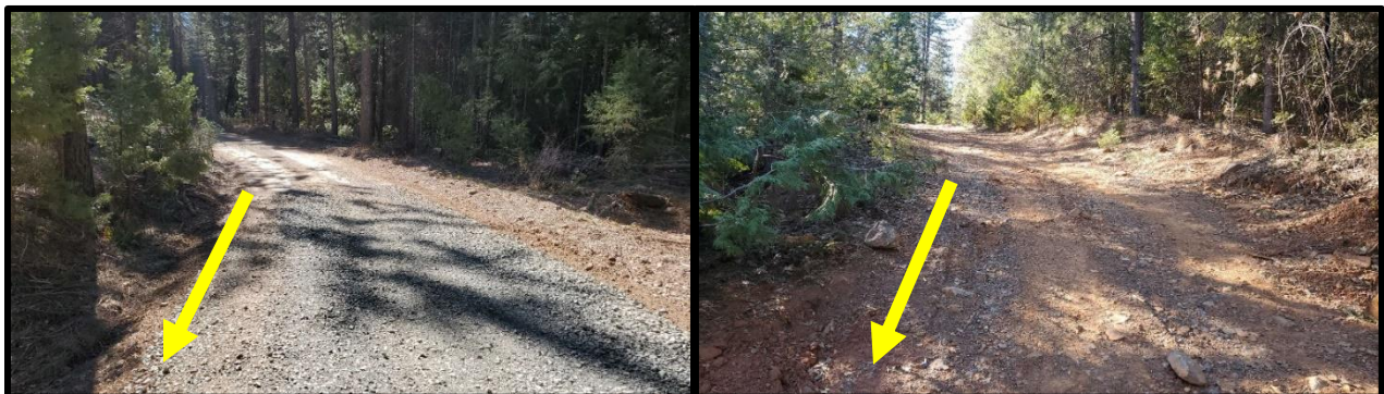
Figure 20: Two examples of approaches to watercourse crossings, with an improved rocked approach (left), and an unimproved native surface approach (right). Yellow arrows indicate direction towards the crossing.
