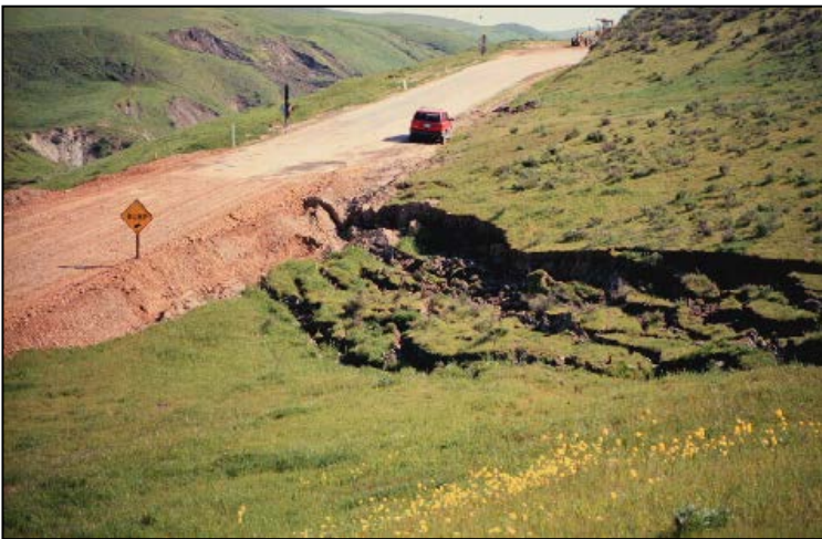
Ground shaking associated with earthquakes can cause slope failures.
