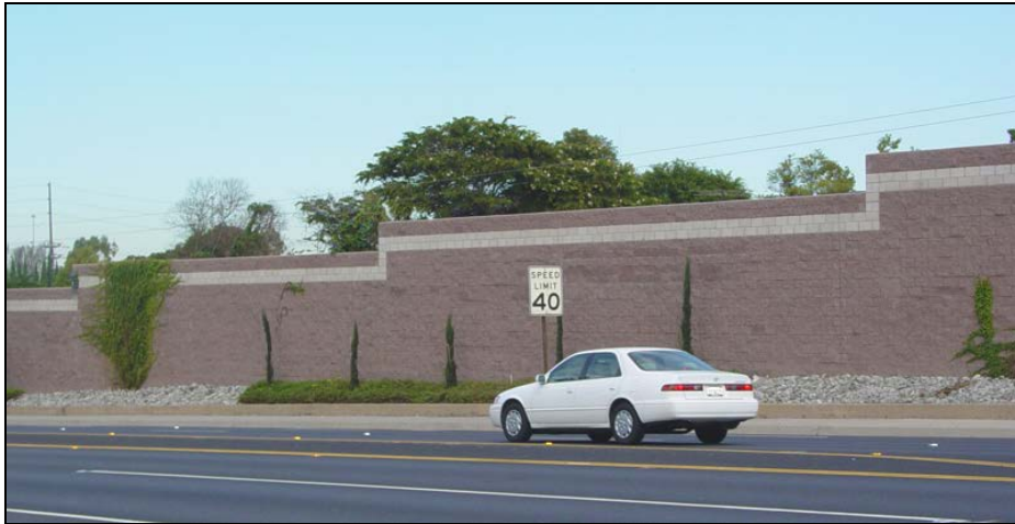
Sound attenuation walls and limits on speed help to shield residential neighborhoods from automobile noise on Imperial Highway.
