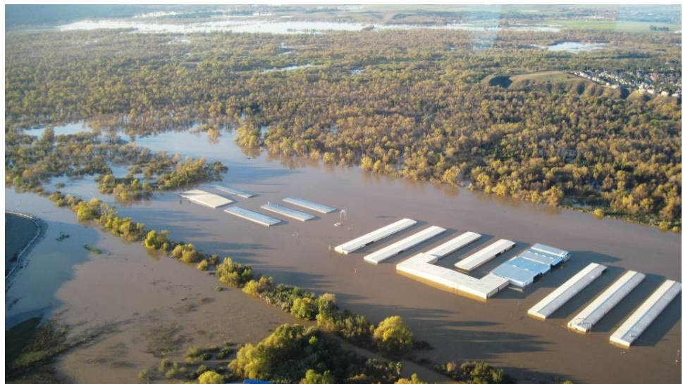
Corona Municipal Airport flooding in 2010, retrieved from http://160knots.com/ .
