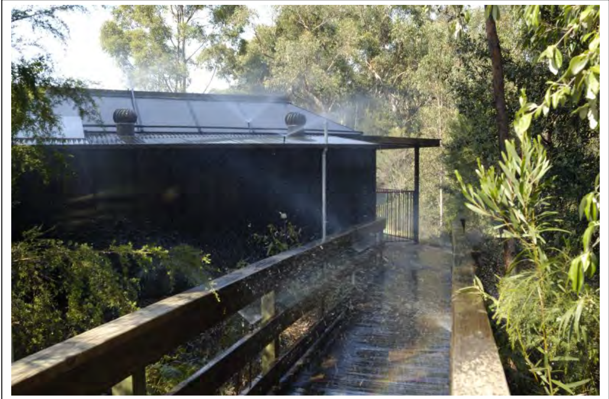
Figure 11. External sprinklers. As a wildfire approaches, external sprinklers wet the structure at risk, the surrounding environment, and increase the local humidity to prevent ignition. Photo: A conference center in New South Wales, Australia.
