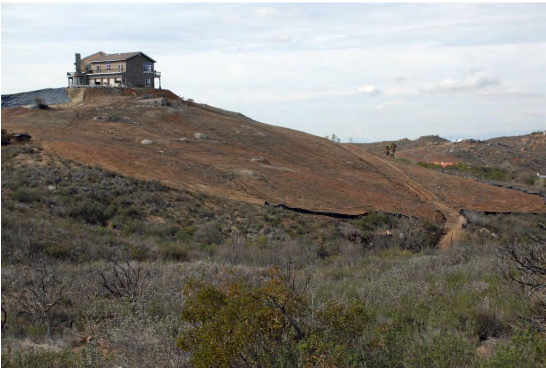
Figure 11. Three-hundred Feet of Clearance. Such bare ground can create a potential “bowling alley” effect, directing embers directly at the structure.
