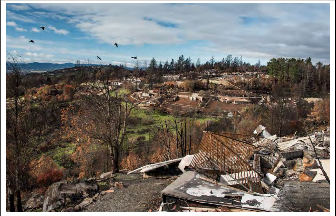
Figure 3. Ridgeline destruction at Fountaingrove II. This photo was taken looking north across the canyon from the former site of the orange-roofed home in the lower right corner of Figure 1.
