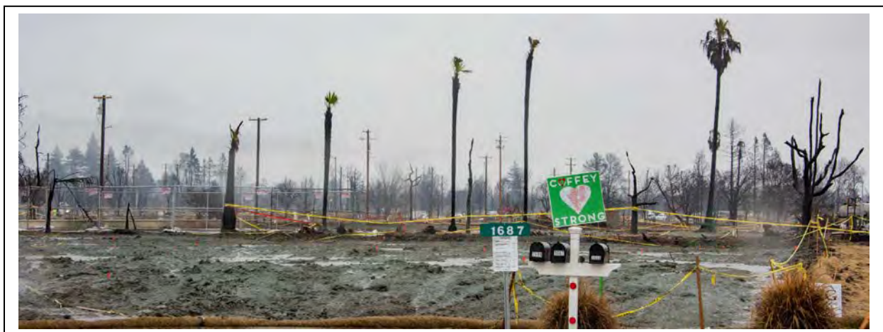
Figure 5: Loss at Coffey Park. An older neighborhood far from the fire front, the entire community was ignited by a massive rain of embers driven by strong winds.
