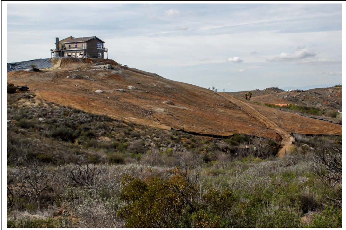
Figure 2 (above). Three-hundred Feet of Clearance. Such bare ground can create a potential “bowling alley” effect, directing embers directly at the structure.
