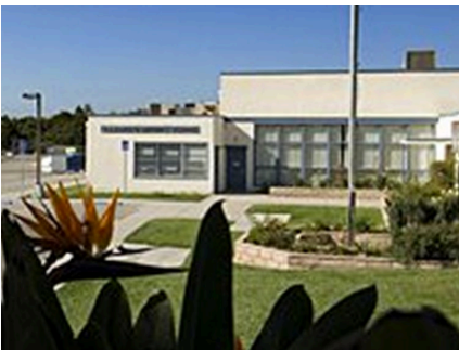
Camarillo Elementary School, Camarillo, CA Remodeling and Addition
