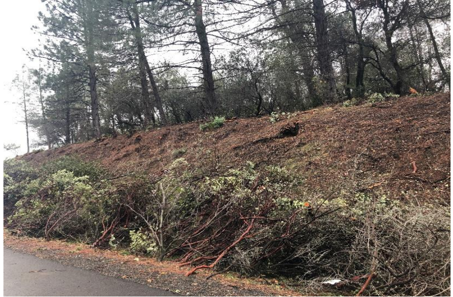
Figure 2-1. Fuel Breaks Underway along Pine Grove Avenue, February 2020. Photo Credit: DP+S
