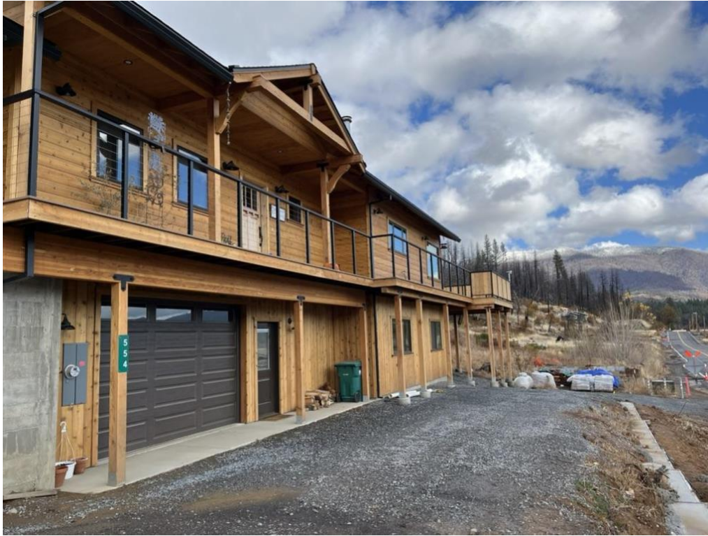
Photo 3. J&C Lumber's cedar lumber featured in the exterior siding of this rebuilt house in downtown Greenville. Photo taken October 2024.
