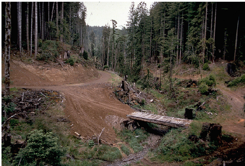
Figure 34. South Fork Caspar Creek roads used in timber harvesting completed from 1971 to 1973. Note native surface roads on both sides of the South Fork watercourse (photo taken in the early 1970s by James Burns, DFG; a similar photo is included in Burns, 1972).
