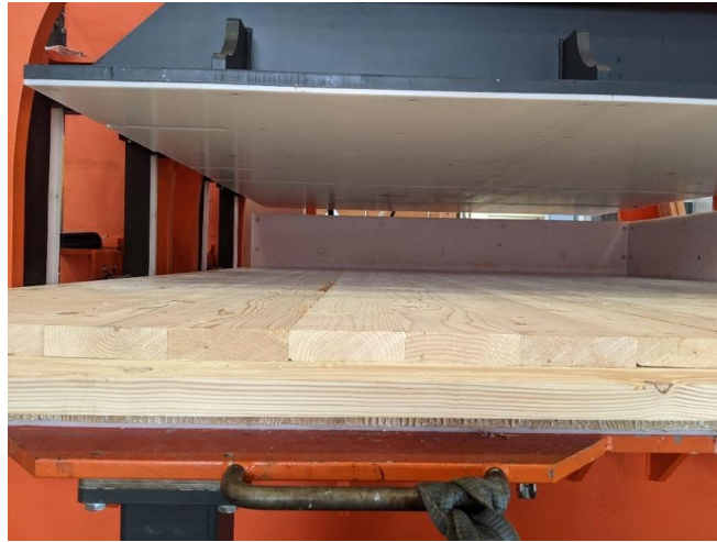
Figure 7: CLT panel immediately after pressing
